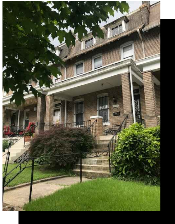
VIEW OF FRONT FACADE
