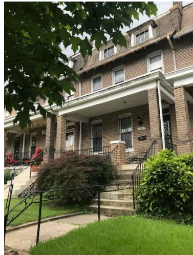
1. VIEW OF EXISTING FRONT FACADE
