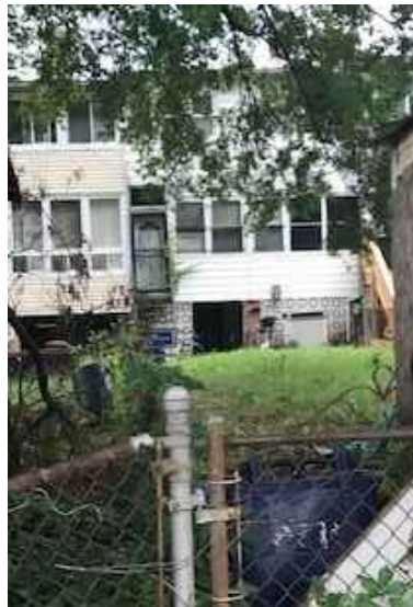
2. VIEW OF EXISTING REAR FACADE
